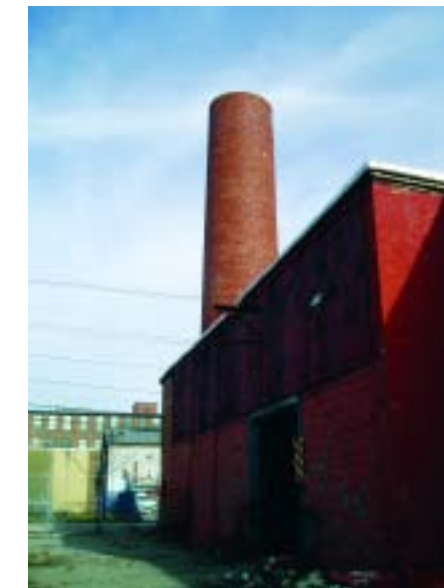
The building and smokestack before the renewal project started.
